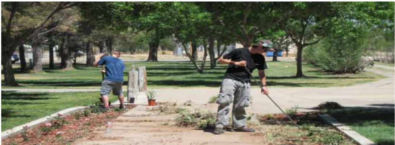
Above: House Municipal School students in New Mexico working on a landscaping project.
