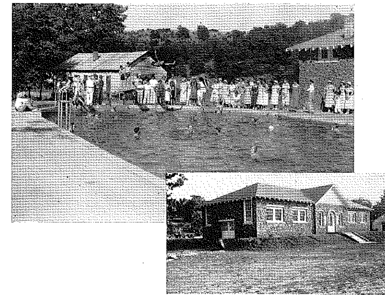
Community Swimming Pool and Farm Shop Building, Sponsored by The Vocational Pupils at Bruno, Arkansas
