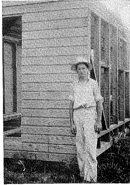
Shop under construction
