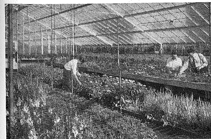
Interior view of the greenhouse which was built by the students in the vocational school. The carpentry work and steelwork was done by students in these departments from material
