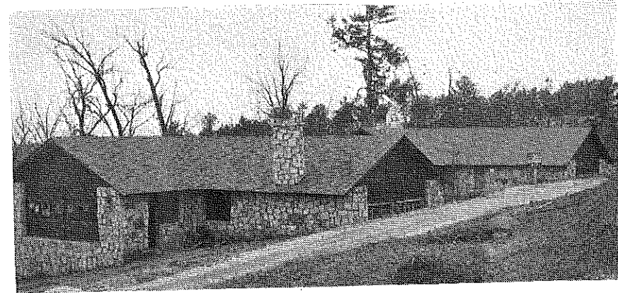
Two large shop buildings where boys are given special training in wood and metal work. The shop will be used during the summer months by teachers of vocational agriculture, who will be given special training in farm shop work
