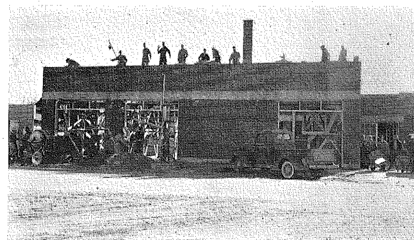
Farm shop class working on new shop building
