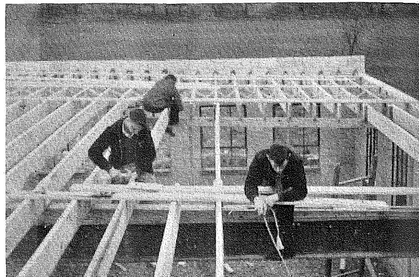
Placing Joists
