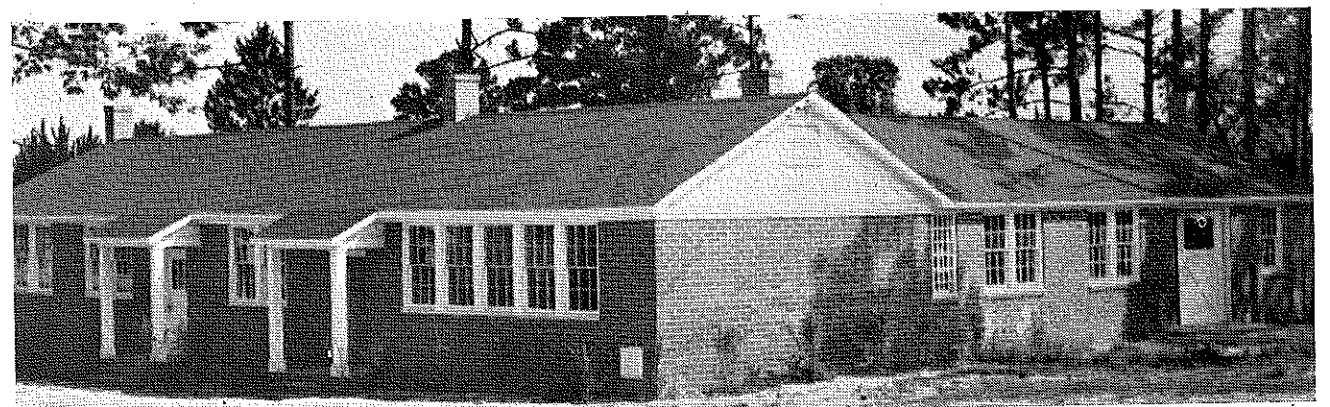
A view of the Swainsboro, Georgia vocational building in which is carried on an extensive program in home economics including a canning kitchen and agriculture including farm mechanics. Education and service are the combined product returned to an appreciative community. S. P. Fugate is the teacher of agriculture, T. G. Walters, the state supervisor
