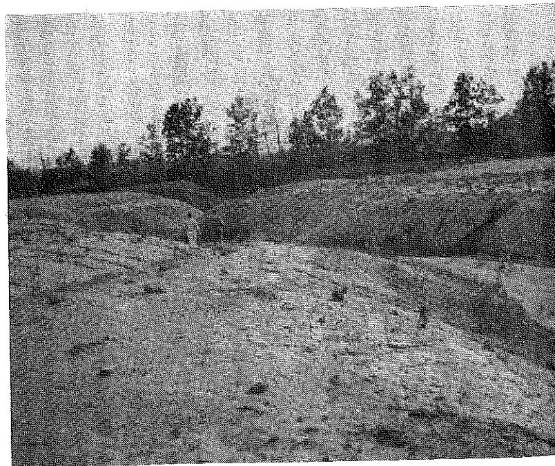
Problems in soil conservation are stressed in the farming programs of students at Sandy Lake, Pennsylvania
