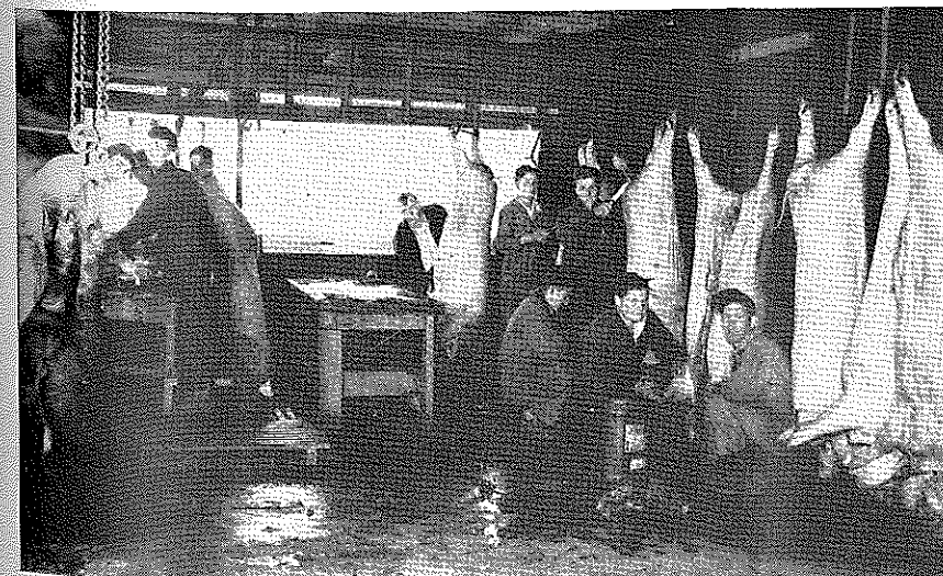
The slaughter house at Rural Retreat is connected by a track to a room in the cannery used for blocking and trimming carcasses.
