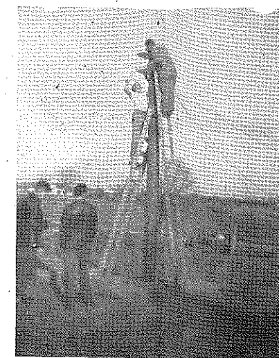
Students installing pole light and three-way switch
