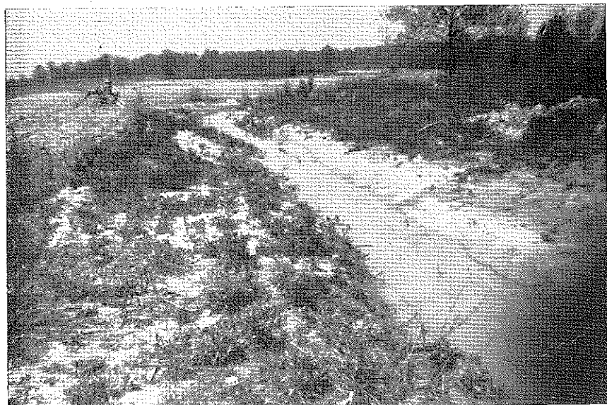
Open ditch drainage project
