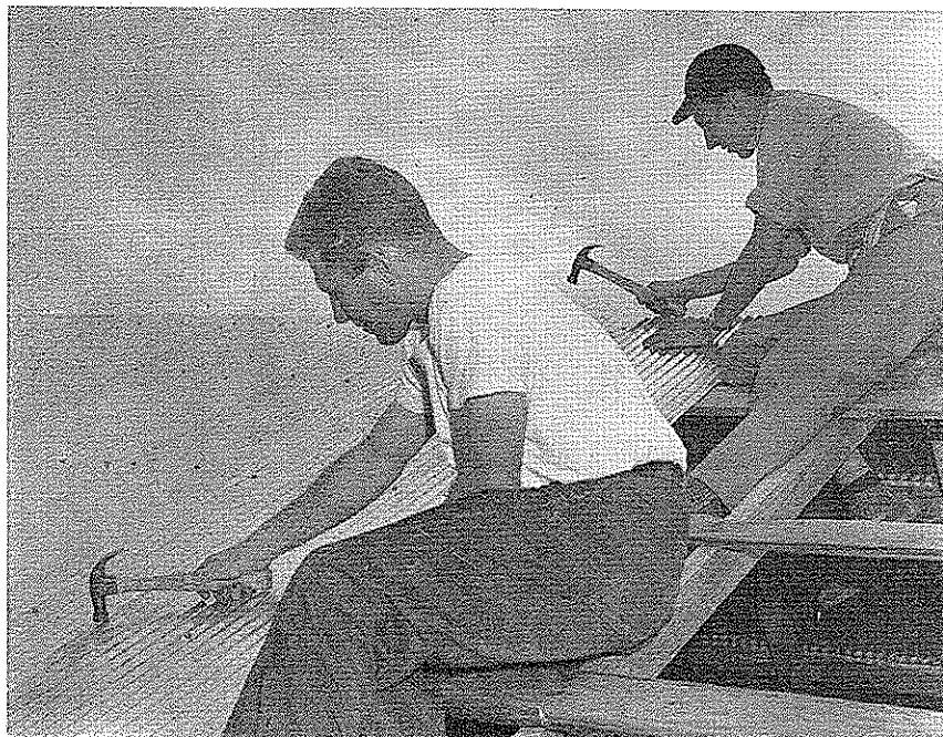
Students apply aluminum roofing find experience beyond class room instruction essential.
