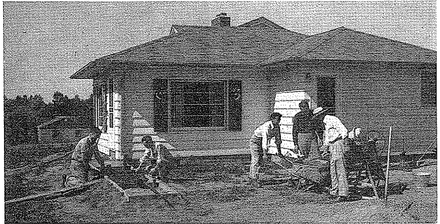
Agriculture instructors framing and pouring concrete for a sidewalk.
