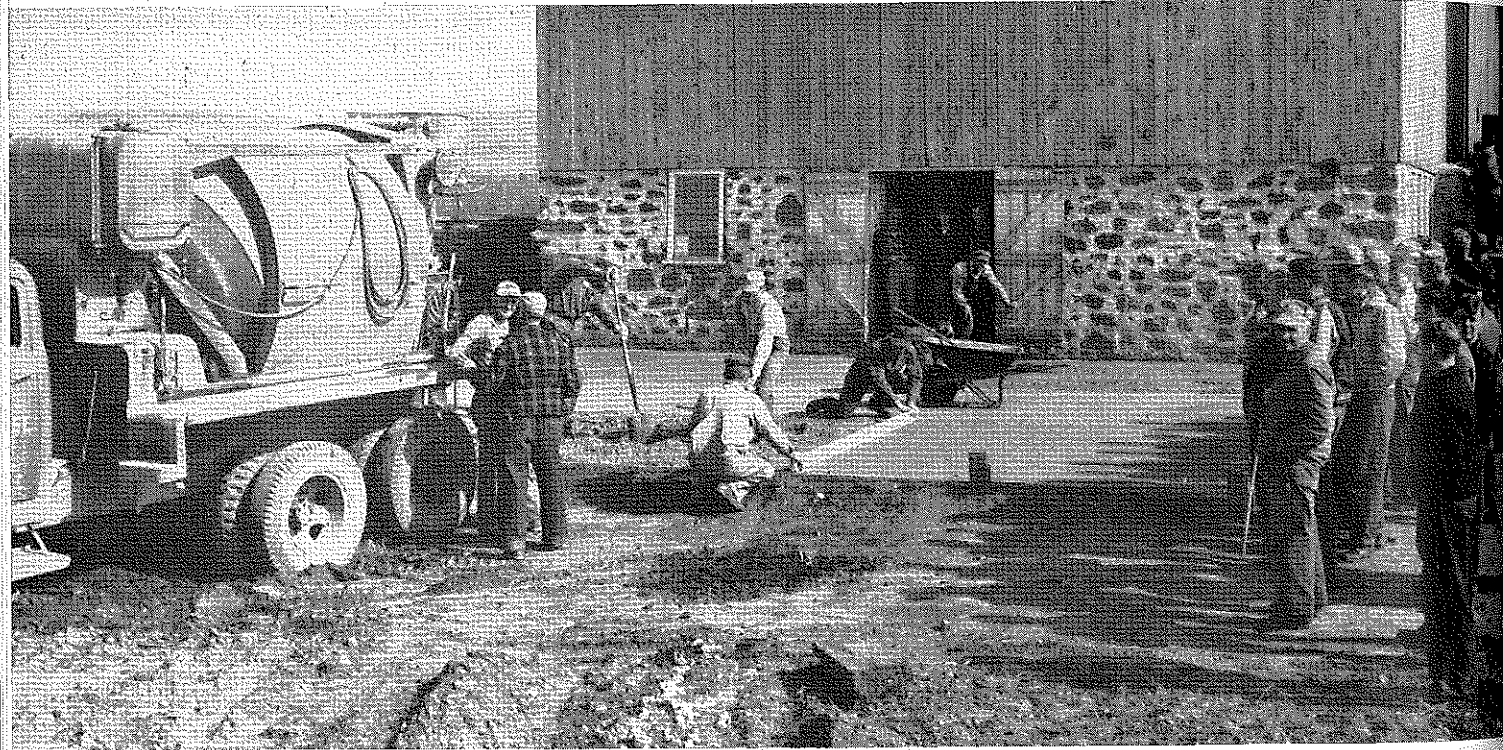
BARNYARD PAVEMENT DEMONSTRATION
