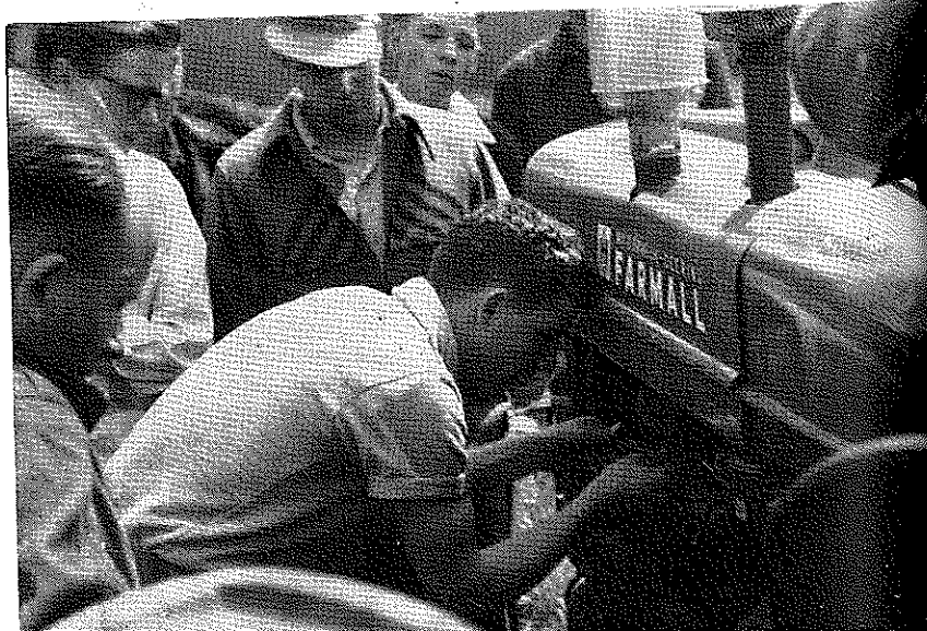
"Adjusting the Carburetor"
