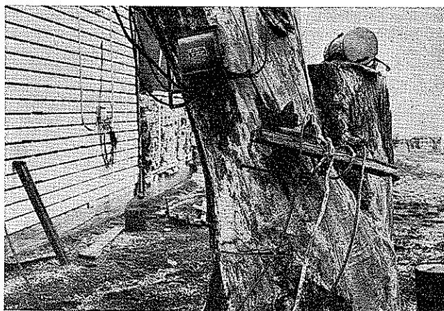
Fig. 4. In contrast to Fig. 3, this shows some actual wiring on a farmstead. These wires were run by inexperienced persons. The crime of such a situation is that on a wet day children can be killed playing around such a set-up.
