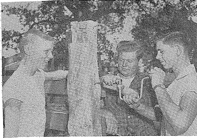
Good gates are very important in farm safety. Here the owner of the farm (center) and classmates construct a new gate as part of the Vo-Ag class work on farm safety.
