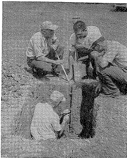
Fig. 1. Shaping the profile slice of soil before applying the metal frame.
