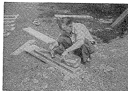
Fig. 4. Impregnating soil profile mount with vinylite resin—first application.
