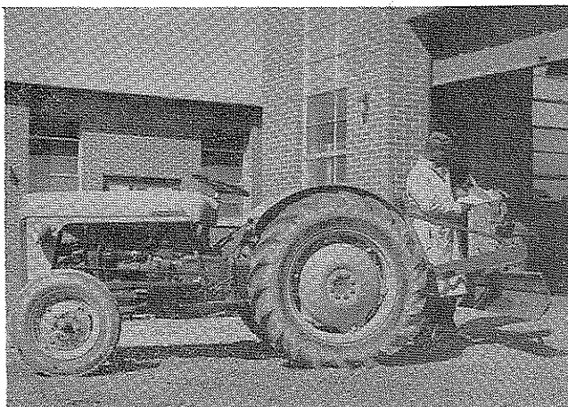
A tractor blade constructed by a young farmer from scrap and discarded materials. It cost this young man only labor, paint and electrodes. A similar blade would retail for $172.00.
