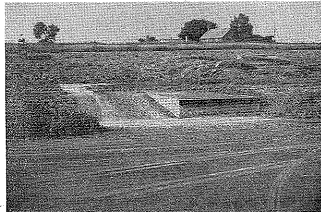
Loading Ramp Suitable for Uneven Topography.
