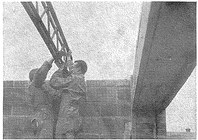
Practice in placing structural steel was provided.
