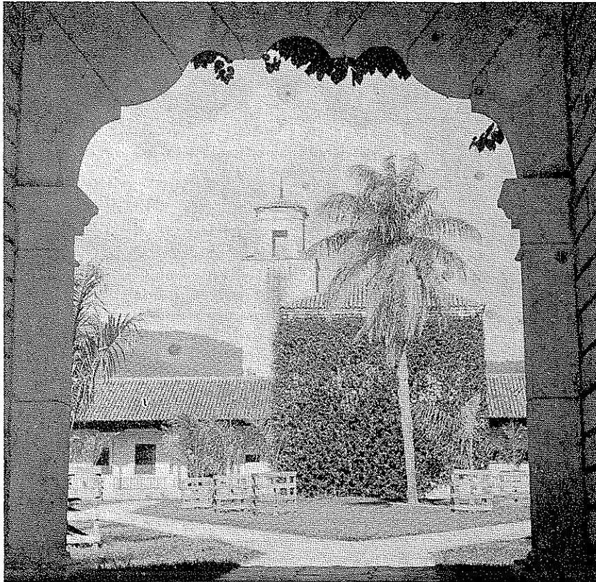
The Administration Building at the Pan American School of Agriculture in Central Honduras.
