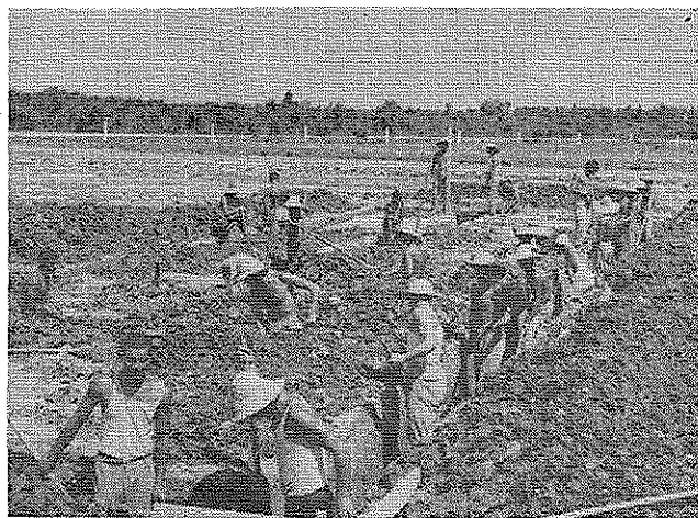
The technician must often work toward gradually combining old ways with new technology as illustrated by the use of traditional hand labor to dig foundation trenches and the use of cement blocks made in a locally built one-man operated block machine. The building under construction is a new school in northern Iran.
