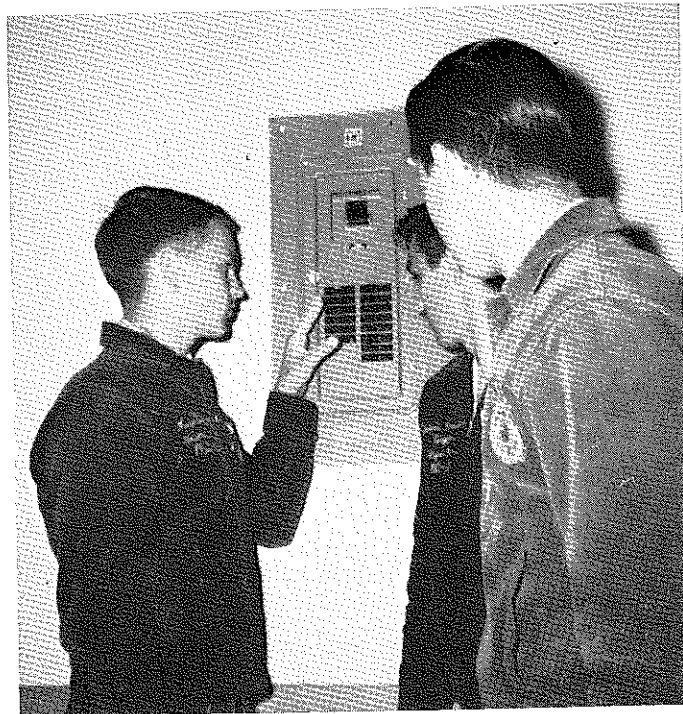
Members become familiar with main electrical switches.
