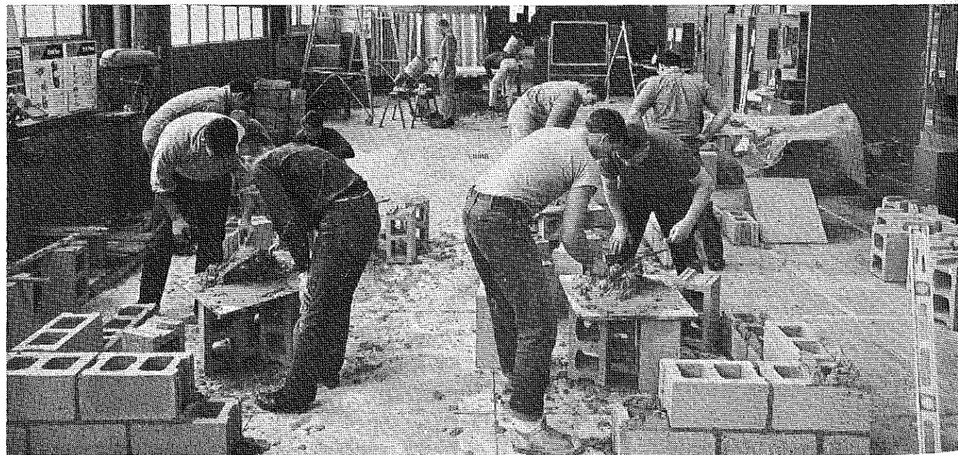
Future Minnesota vocational agriculture teachers, enrolled in Methods of Teaching Agricultural Mechanics, learn concrete block construction principles by the "doing process." (Photo by F. Bear)
