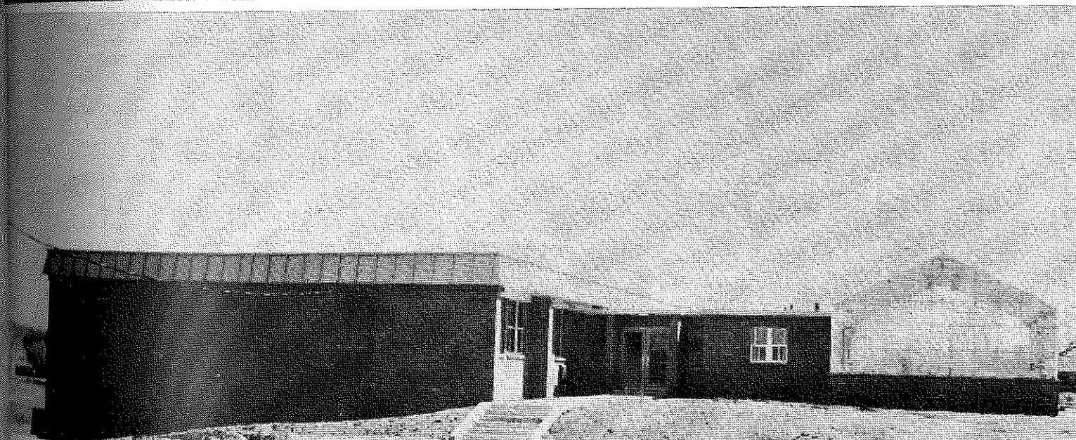
Innovative programs in Maryland's Vocational Agriculture departments include facilities for Greenhouse management, separate library, and the applied science research laboratory.
