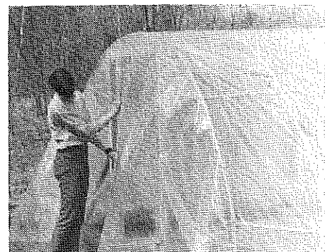
Polyethylene plastic is easily drawn over the structure and fastened to the wood foundation along the sides and ends of the greenhouse with lath. The plastic is lathed to the framing on the ends. Excess plastic at the corners is rolled tightly and fastened to the wood foundation.
