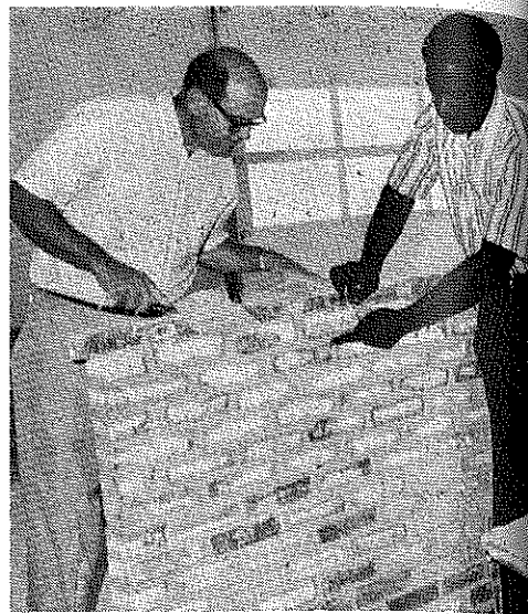
Individual instruction is provided in this Masonry Workshop.
