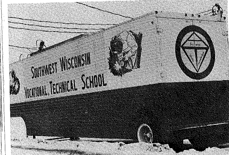
This 37 foot long mobile welding trailer, owned by the Southwest Wisconsin Vocational-Technical School, is transported to various locations in the five-county district. The trailer can accommodate eight arc and oxy-acetylene welders and four M.I.G. and T.I.G. units simultaneously. Inside the mobile welding unit, a Production Agriculture student is busy practicing stick-electrode welding techniques. The trailer contains its own power, storage space, and heating and ventilating units. (Photos from John F. McNeill, Supervisor of Production Agriculture, Fennimore, Wisconsin).
