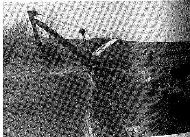
DITCHING —Improving and maintaining the soil is an integral part of the instruction in natural resources. Here a ditcher is observed operating on the E. V. King Ranch, Silverton, Oregon. (Photo from Rodney Tulloch, University of Kentucky, and U.S. Department of Agriculture)
