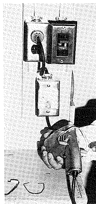
PHOTO 1 Patch cords with varying degrees of resistance for plugging into drill handle.
