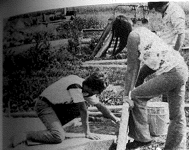
A landscape construction class builds a patio.
