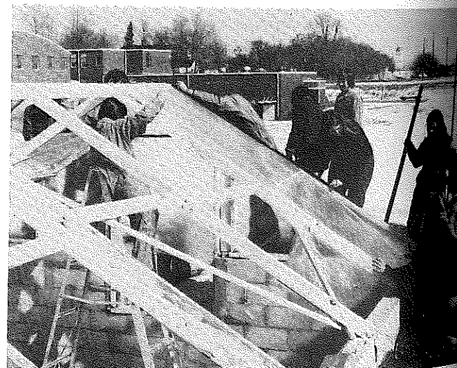
Students covering sash house. It is used to grow most all types of plants and is heated only by the sun.
