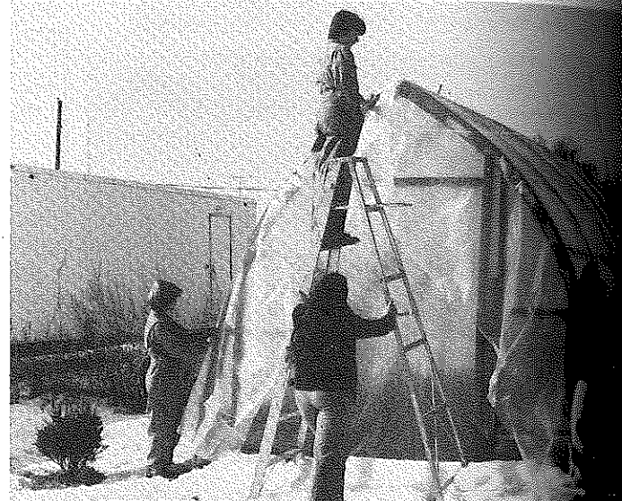
Students at Bath County High School, Owingsville, KY, cover a greenhouse with plastic for use with geraniums in the spring. (Photo courtesy Jimmie Watson, Bath Co. H.S. Related story on p. 142)
