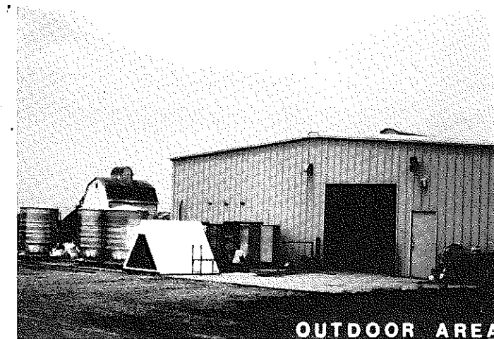
Figure 3. Outdoor Area — provide 2100 sq. ft. of area adjacent to the Ag Mech. Lab. for approved project work; at least 1500 sq. ft. of the area should be hardsurfaced and 500 sq. ft. roofed. A fence or wall would provide security and is aesthetically more pleasing.
