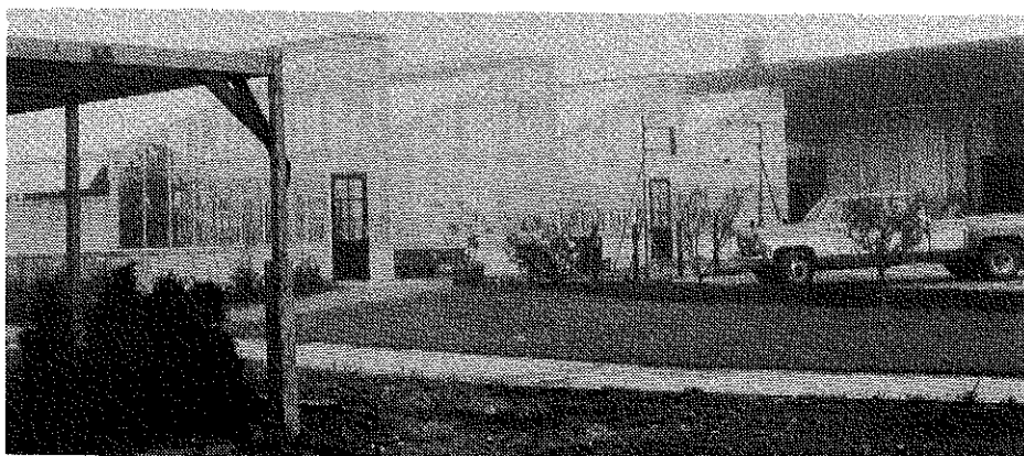
The greenhouse facilities include 8,500 square feet of floor area.
