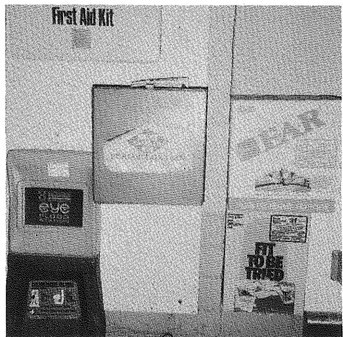
Personal safety equipment and first aid equipment must be grouped for easy access and use by students. Safety equipment must include hearing protection devices.
