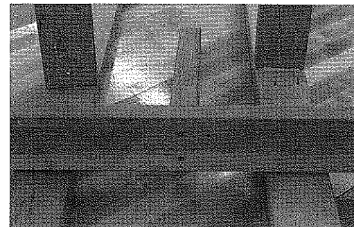
Photo 1. 2 x 4 studs fastened with glue, 16 penny nails, and 8 penny nails. (Photo courtesy of Glen M. Miller.)
