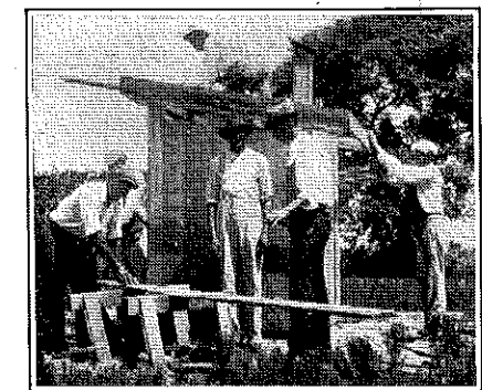
Sanitary toilets were built.
