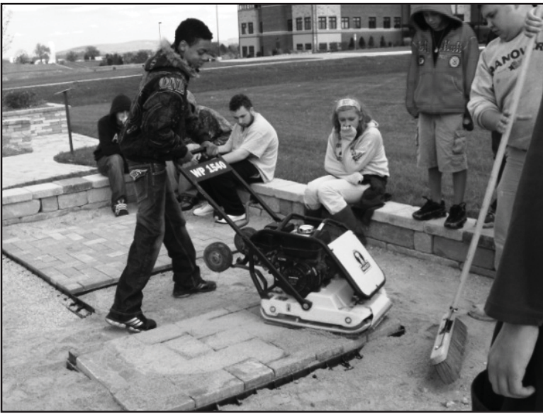
Gettysburg Area High School students compacting pavers.
