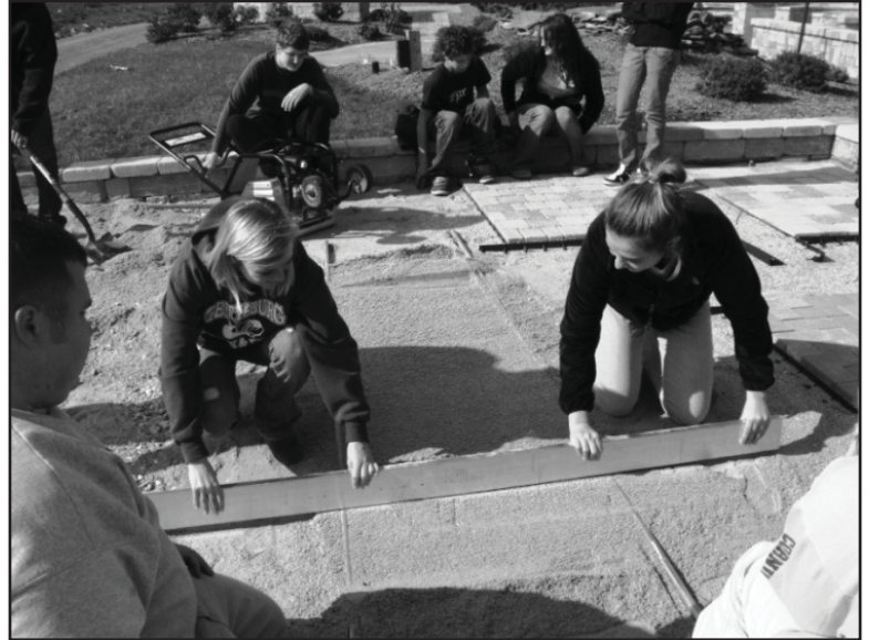
Gettysburg Area High School students screening sand before placing pavers.
