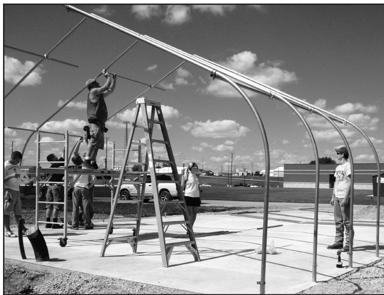
Students constructing a greenhouse with a 180 spot hydroponics system.
